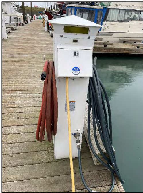
Figure 2.55: Electrical power service pedestals on EE Float (left) and typical of HH & JJ Floats (right). Note that the newer pedestal also incorporates water hose bibs.
