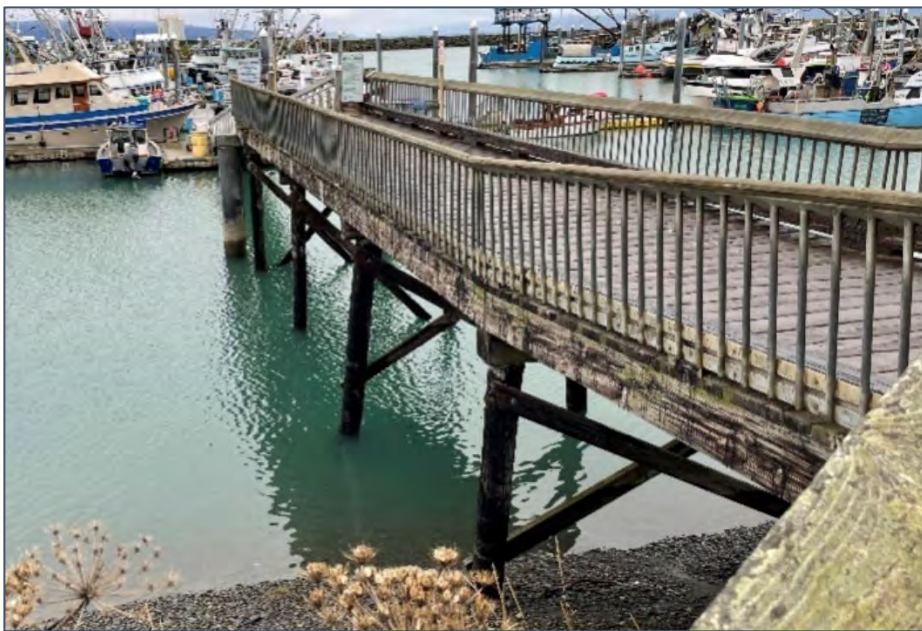
Figure 2.2: Ramp 1 timber pile supported trestle.
