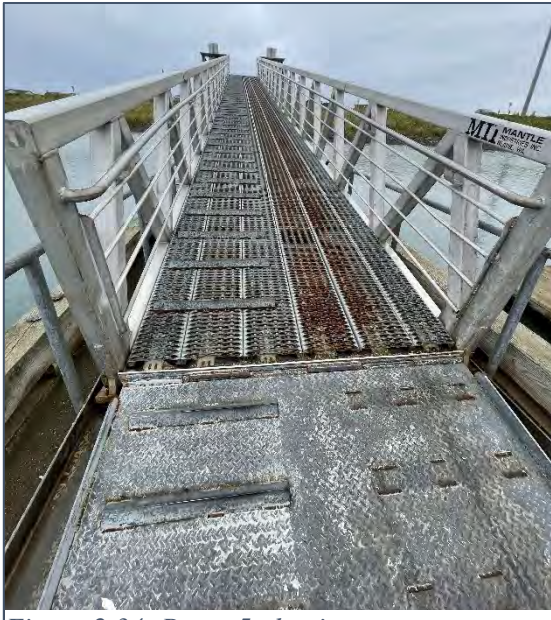
Figure 2.34: Ramp 5 aluminum gangway w steel floor grating.
