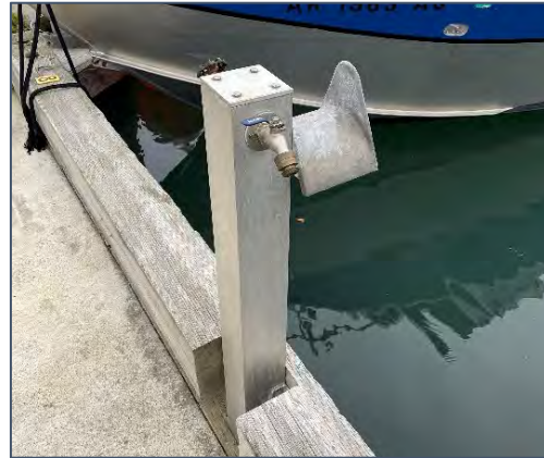
Figure 2.42: water hose bib and hose stand.
