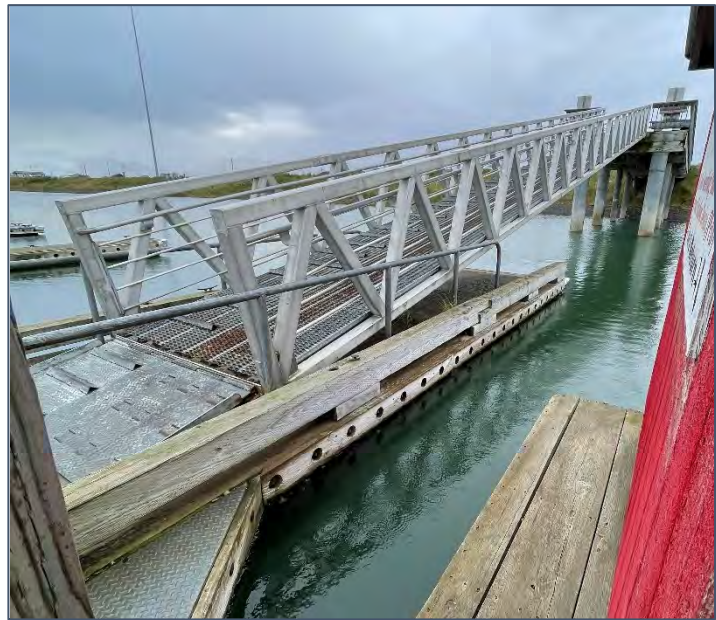
Figure 2.35: Ramp 5 trestle and gangway. Note landing on concrete float with reduced freeboard.
