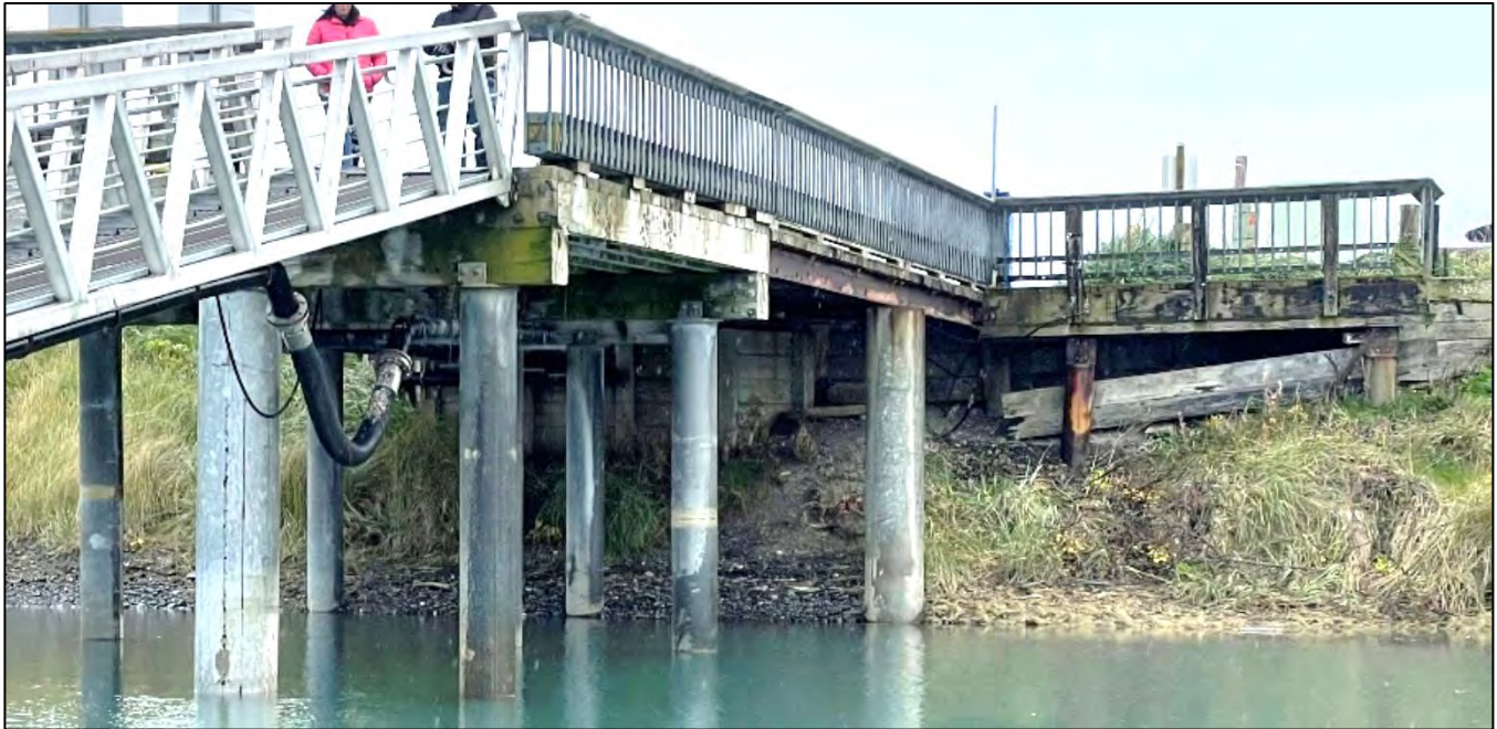
Figure 2.8: Ramp 4 trestle, noting newer/older portions of timber trestle and pile-to-beam attachments.
