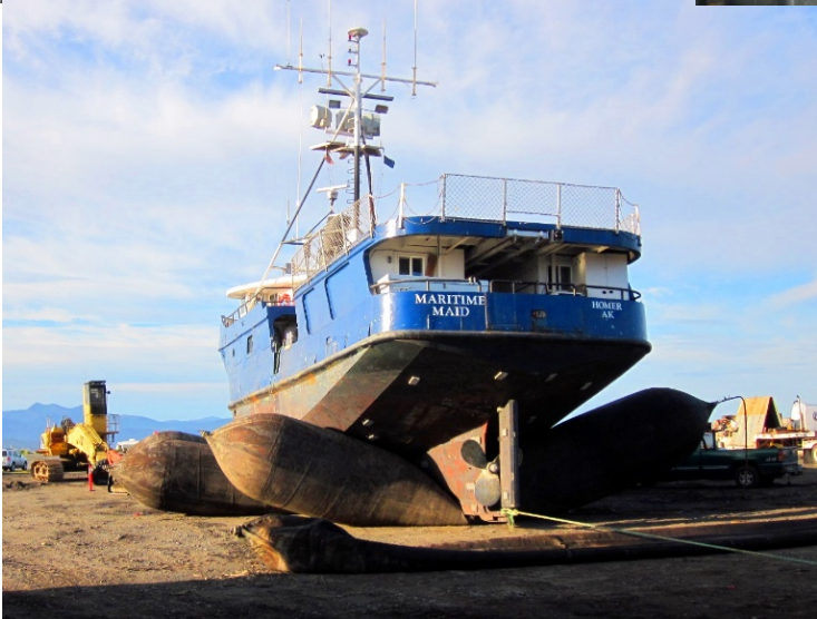
Pictured: Concrete Pouring For Boathouse Pavilion, Maritime Maid Haul Out, New LED Lighting For High Mast Lights
