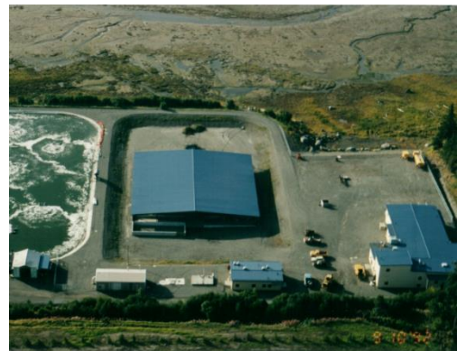
Sewer Treatment Plant (1990)
