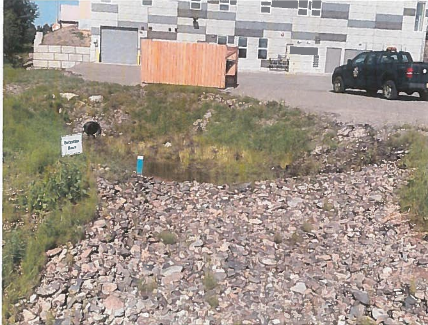
New Storm Water DETENTION BASIN - site runoff directed to basin - peak runoff from the site reduced to pre-construction levels
