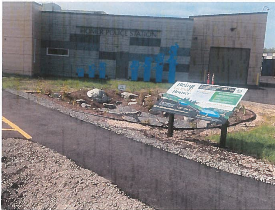
New RAIN GARDEN - site drainage directed to garden to slow peak storm water and filter sediments
