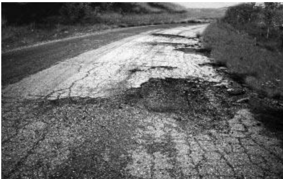
◀ Large, isolated pothole, extends through base.
