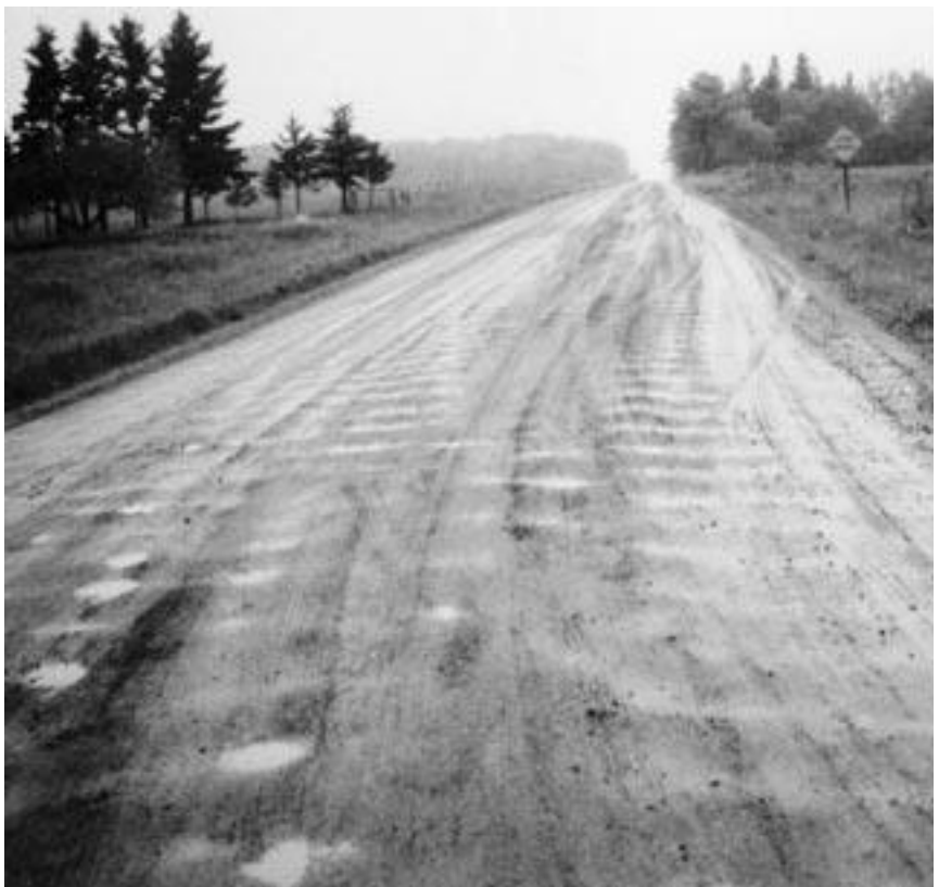
► Severe washboarding traps water.
