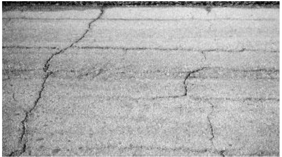
▼ Block cracking with open cracks.
